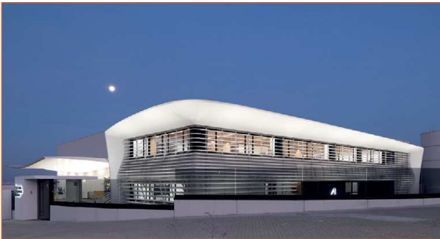
Fig. 4: General view of the installed composite elements in the building
