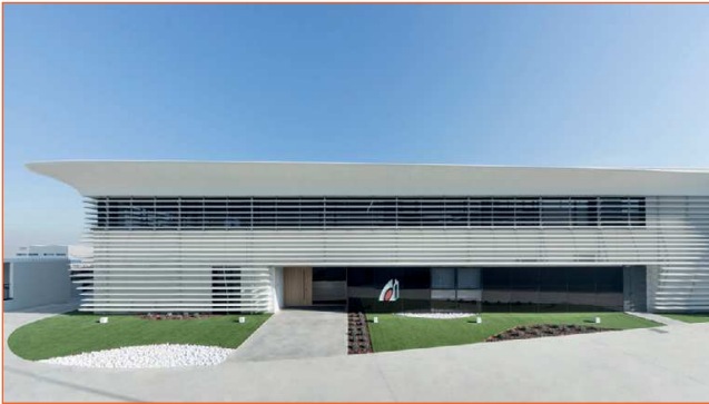
Fig. 3: General view of the office block, showing The White Bow
